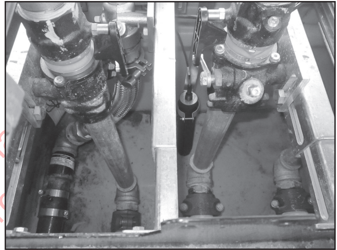
FIGURE 8-3. The sensor needs to be properly positioned to detect the presence of liquid in sumps.
