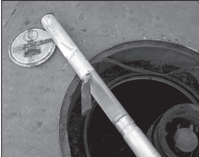
FIGURE 7-1. Check the drop tube and flapper for damage. Make sure that the flapper moves freely and will move into the product flow path.
